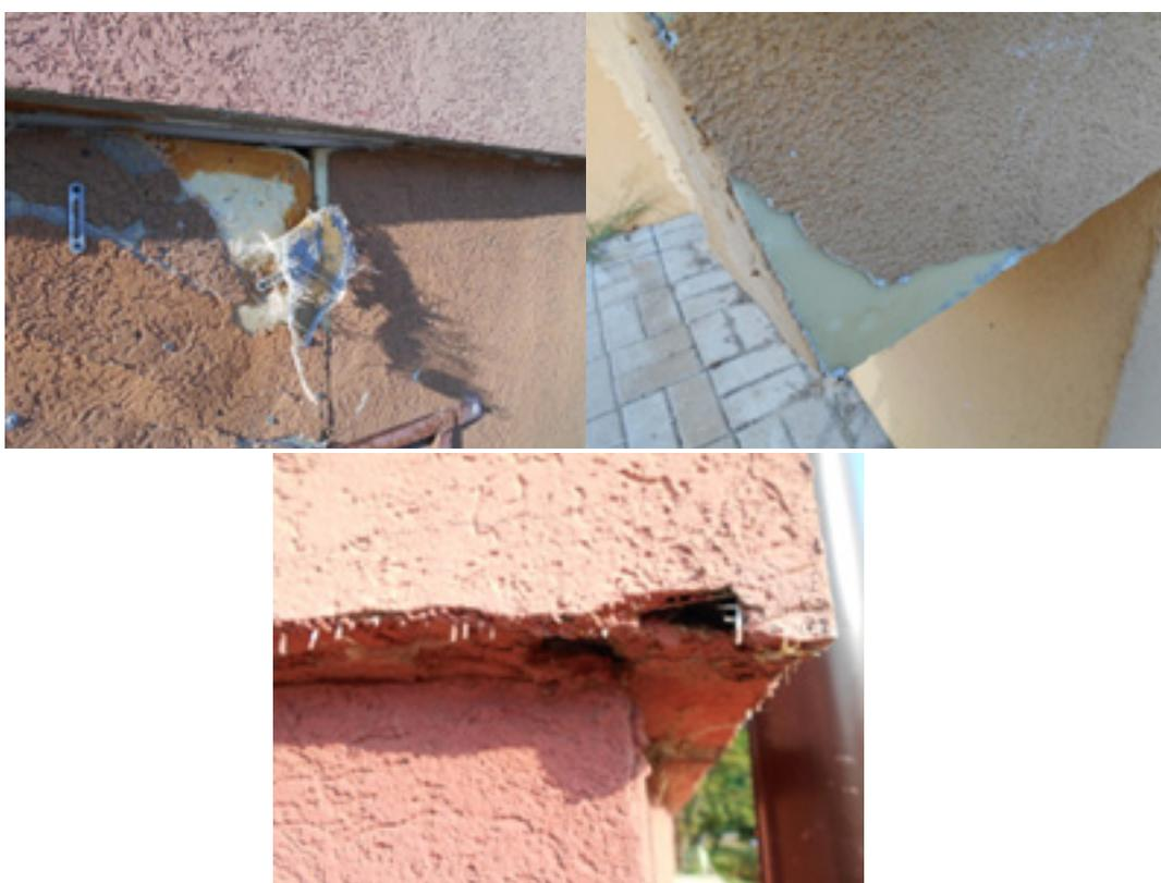
Figure 1. Defects in the installation of glass-fibre wrapping material under the plaster base.
