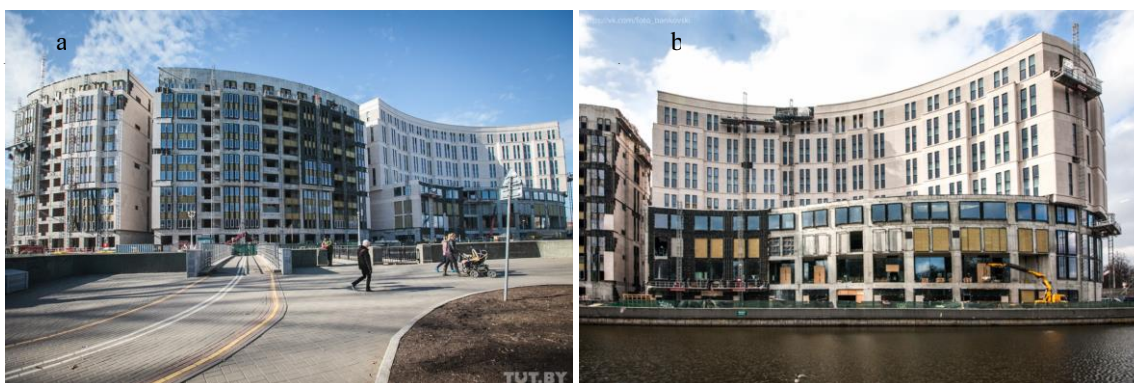
Figure 8. A multifunctional complex with the Kempinski hotel as of 2014 [6]: a) view from the street. Y. Kupala; b) view from the side of the river Svisloch
