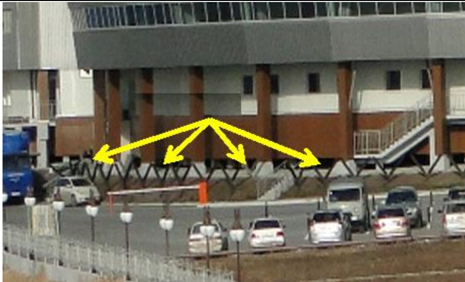
Fig. 2. The location of the seasonally operating cooling devices.
